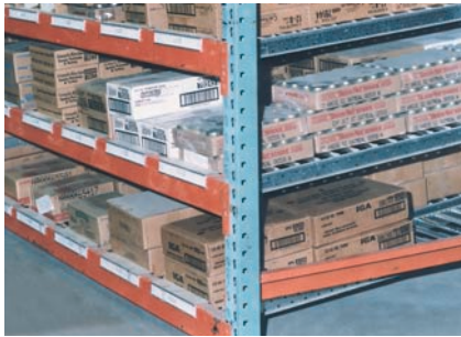
Low Profile Span-Track Track “nests” between beams.
