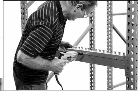
Retainer angle installs on top outside (aisle side) edge of front and rear beams
